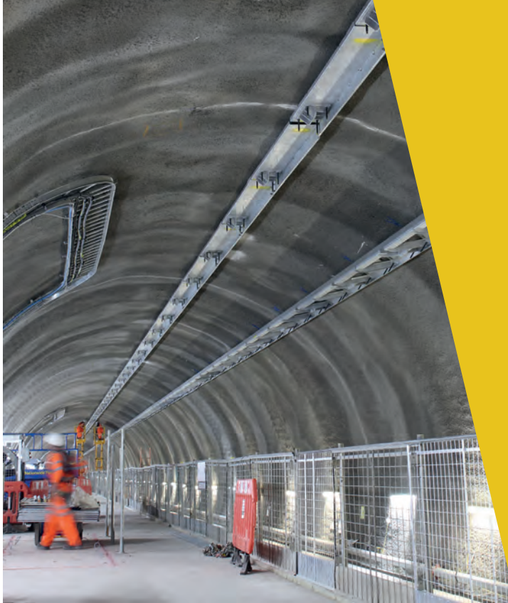
Crossrail, Tottenham Court Road PLUS Bolt installations
